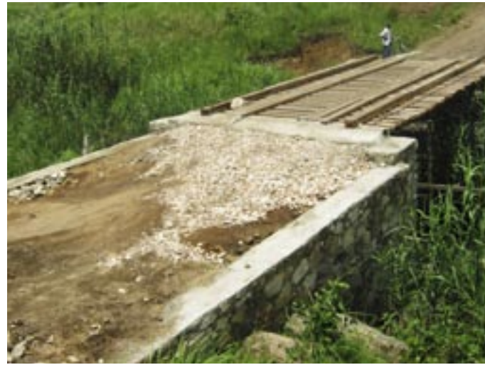
The cement bridge will make it easier to get to services all year around Bembeyi, Meso Ulola, 2009
