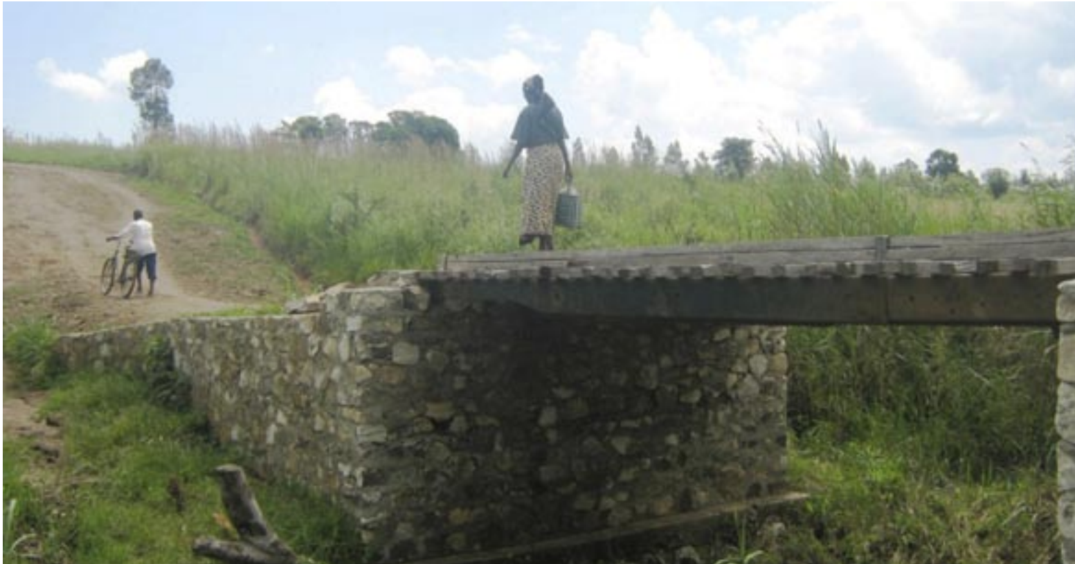
Several months in the year we couldn't reach the health centre when the river flooded. So we made a plan to change the wooden bridge to a durable stone and cement bridge. Bembeyi, Meso Ulola, 2009
