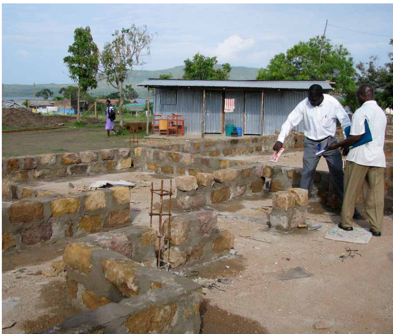
Building work underway on new maternity wing for Mbita sub-district Hospital, Nyanza province, Kenya
