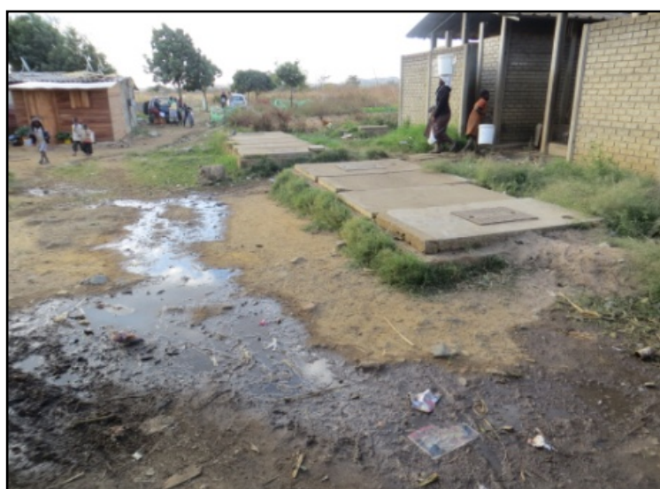
Burst sewer pipe close to the ablution block, TARSC 2014
